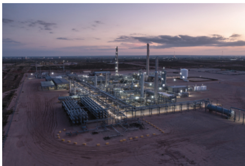
Carlsbad Processing Plant acquired from Sendero Midstream in July 2022
